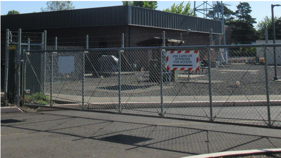
Looking NE at site entrance with dumpster enclosure (left) and development area (right).
