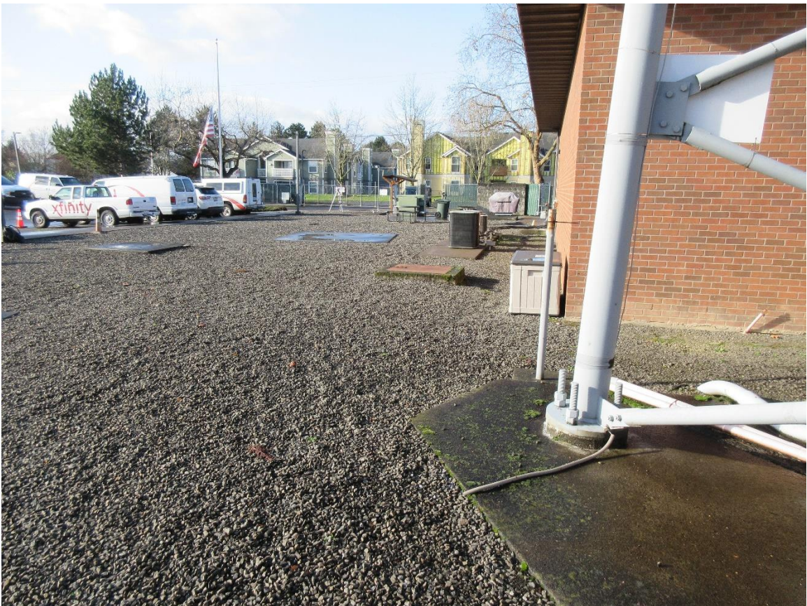
Looking west at existing gravel area for replacement generator units.
