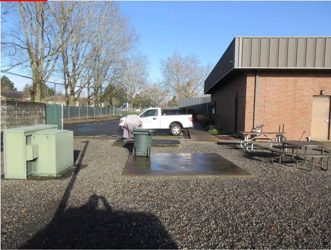
Looking north at dumpster enclosure (left) and part of building (right).
